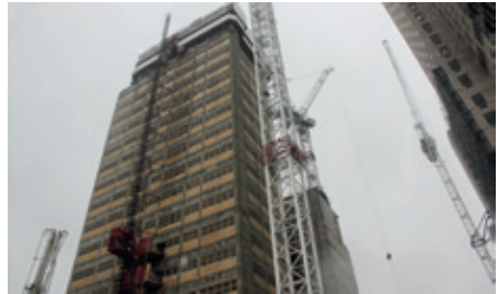
A new look for One Southbank Place
